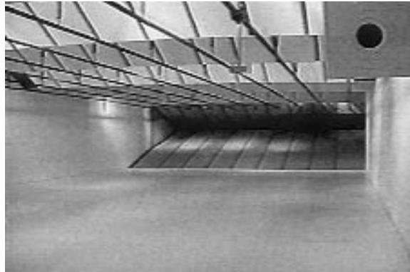
*This backstop consists of gentle sloped metal impact plates which direct projectiles into a collection chamber. Cost of installation is moderate to high. It can handle all calibers up to and including .50. It is durable, reduces bullet fragmentation and lead dust, and projectile collection is relatively easy.*
